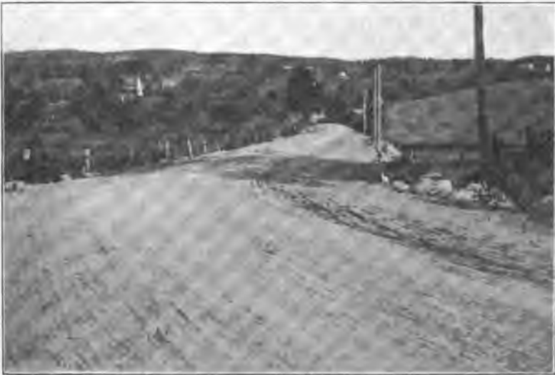
Stanhope and Newton road, Sussex Co., after improvement.
